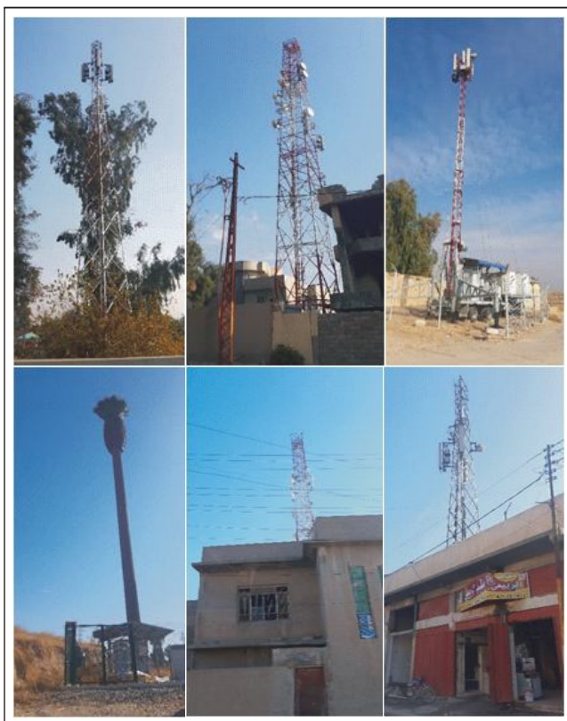
Fig. 3: Shows different types of antenna structures found in the survey.
