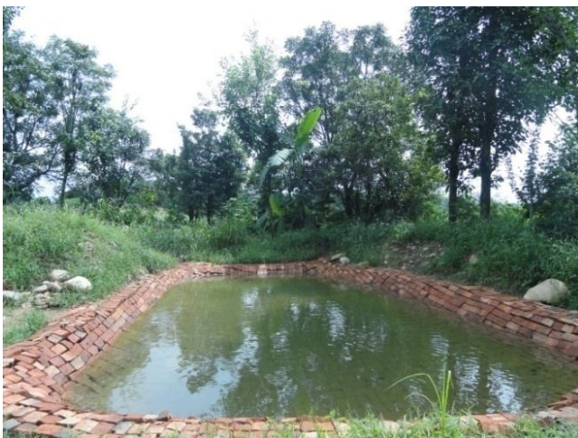
Fig. 2: Polylined tank Rain Water Harvesting Technique.
