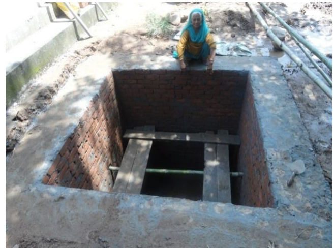
Fig. 3: RCC Tank/Roof Rain Water Harvesting Technique.
