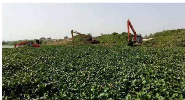
Mechanical pulling out of Nile flower plant widely spread in the Iraqi rivers
